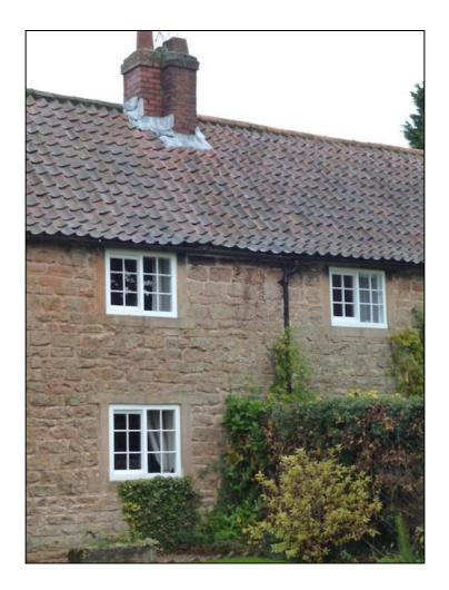
**Photo 21:** Details of local construction methods and materials, at nos. 67-73, Main Street, illustrate the use of local magnesian limestone with a pantile roofs and Yorkshire (horizontal) sliding sash windows
